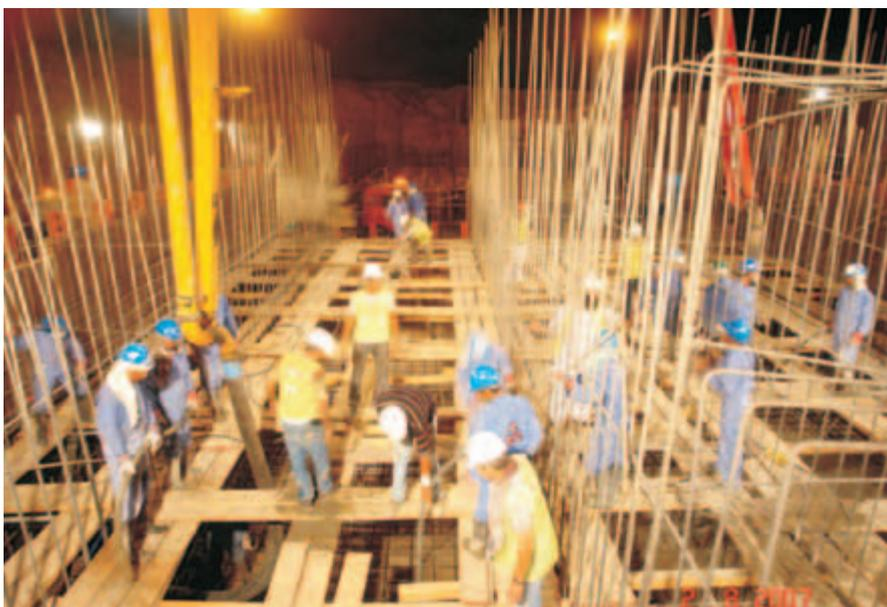
◀ *Pouring concrete at night to avoid the high temperature during the day.*
