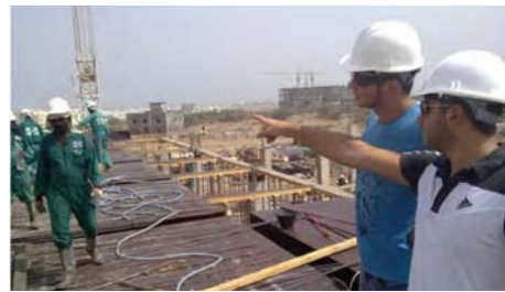
❖ Carl Abi Saab (Electrical Engineer on the right) and Hanna Abi Saab (Civil Engineer next to him) at Bawshar site near the capital Muscat. Concreting of roof and installation of electrical conduits.
