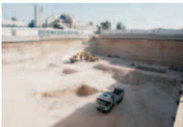
Excavations of the Abdali Project
