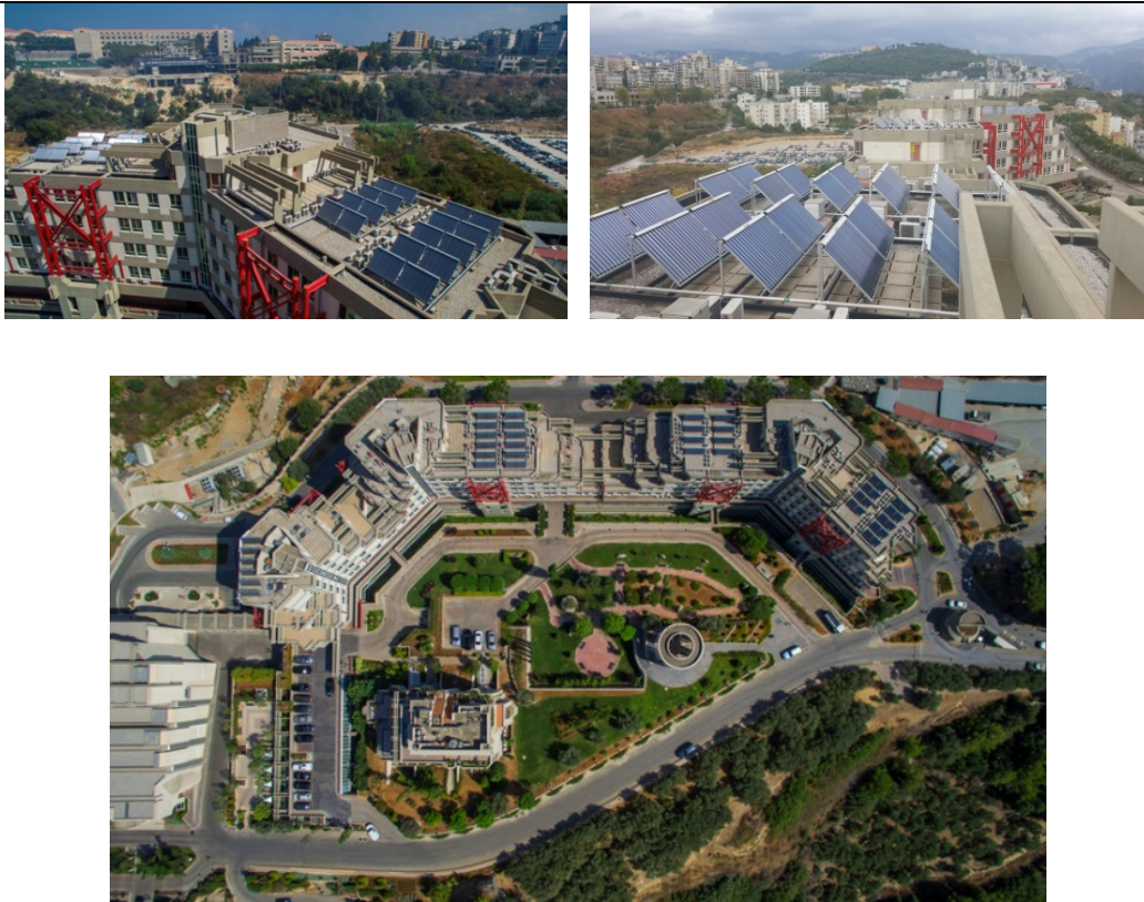
Solar Water Heating System Installed over All Dormitory Buildings
