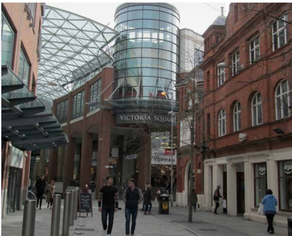
Figure 2: A postmodern shopping experience under the dome of Victoria Square, Belfast.
