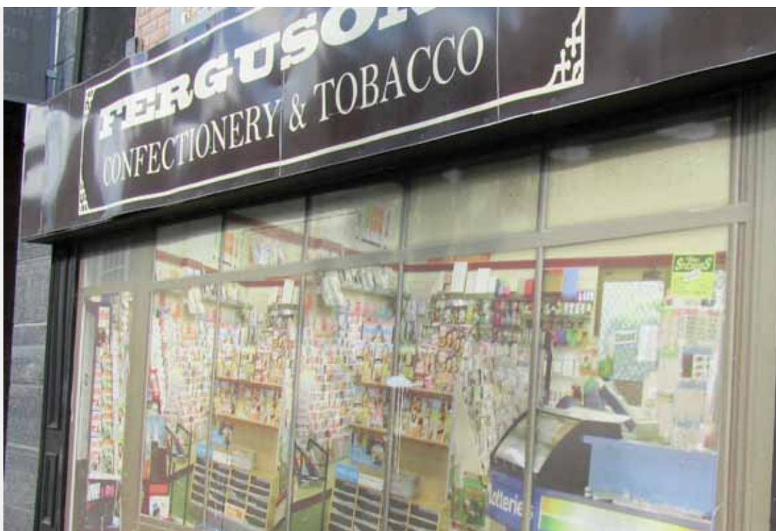
Figure 17: Fake Fergusons confectionery and tobacco shop, with its now buckled metal fascia board
