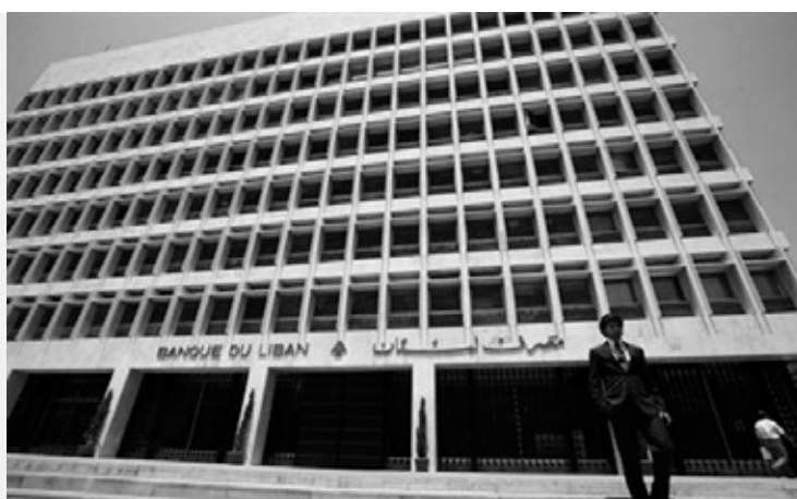
Fig 2. The Central Bank Building in Hamra. 1970's [Online] Lebanese Embassy in Stockholm.
