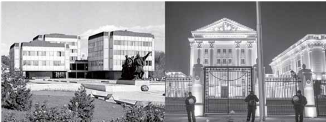
Figure 4: . Building of the central government of Republic of Macedonia before the transformation (left) and after (right)
