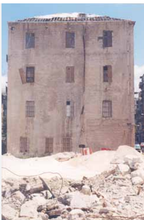
Figure 4: Landmark Beiruti House on Lot 581 prior to renovation. The building's secondary façade now faces the main avenue. Source: Fouad Menem Architects.
