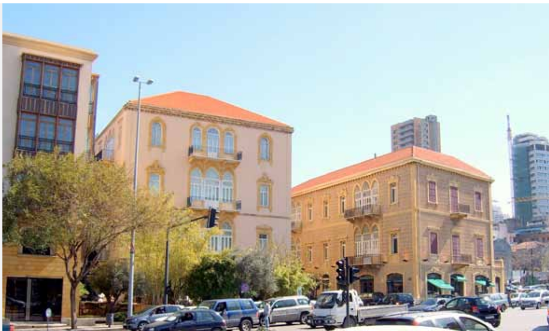
Figure 5: Lot 581 after renovation (building in the middle of the picture) now houses a French café-bistro with 4 residential units in the upper floors. In contrast with the former picture, the main façade is now facing Georges Haddad Avenue. Source: the Author
