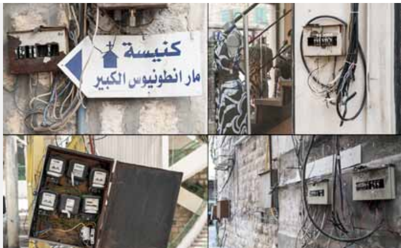
Figure 1: Circuit breakers (disjoncteurs) as they appear on the streets.
