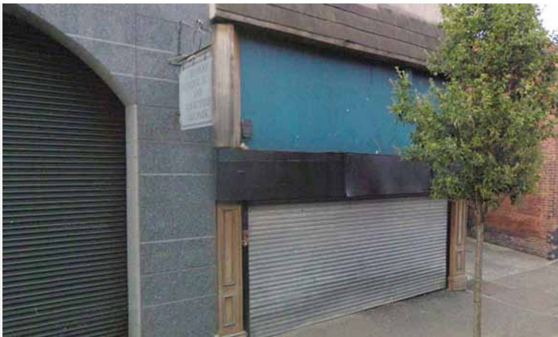
Figure 16: The vacant corner shop, now the location of Fergusons Tobacco fake shopfront
