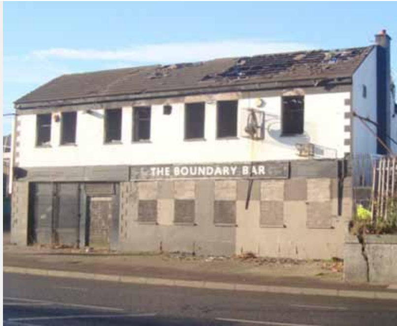
Figure 4: The Boundary Bar, Shore Road, Belfast, before cosmetic treatment
