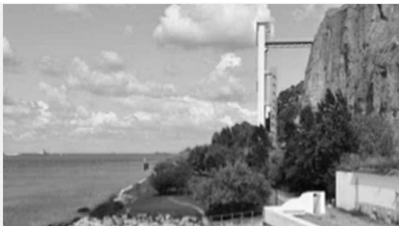
Figure 3: Boca do Vento Lift
