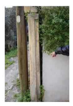
Figure 2: Slope failure, detached retaining wall
